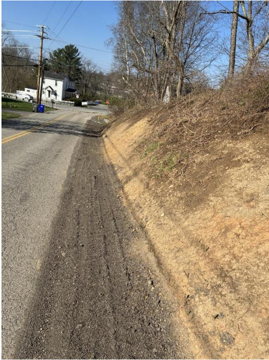
Photograph: Completed phase of work on Marburger Road (2026)
